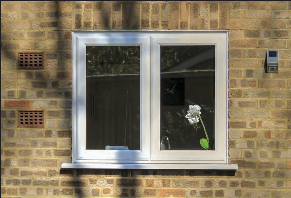
The floating central mullion allows the windows to benefit from the maximum opening without the obstruction of a fixed vertical frame between the opening sashes
