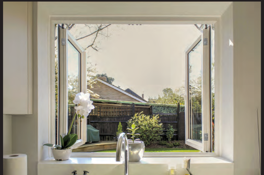
The floating central mullion allows the windows to benefit from the maximum opening without the obstruction of a fixed vertical frame between the opening sashes
