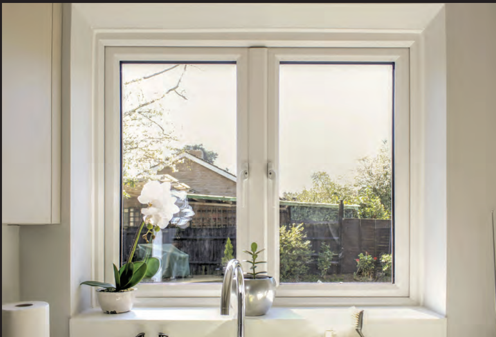
The floating central mullion allows the windows to benefit from the maximum opening without the obstruction of a fixed vertical frame between the opening sashes
