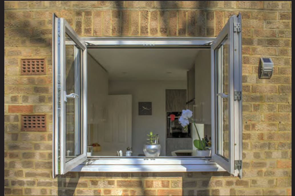
The floating central mullion allows the windows to benefit from the maximum opening without the obstruction of a fixed vertical frame between the opening sashes
