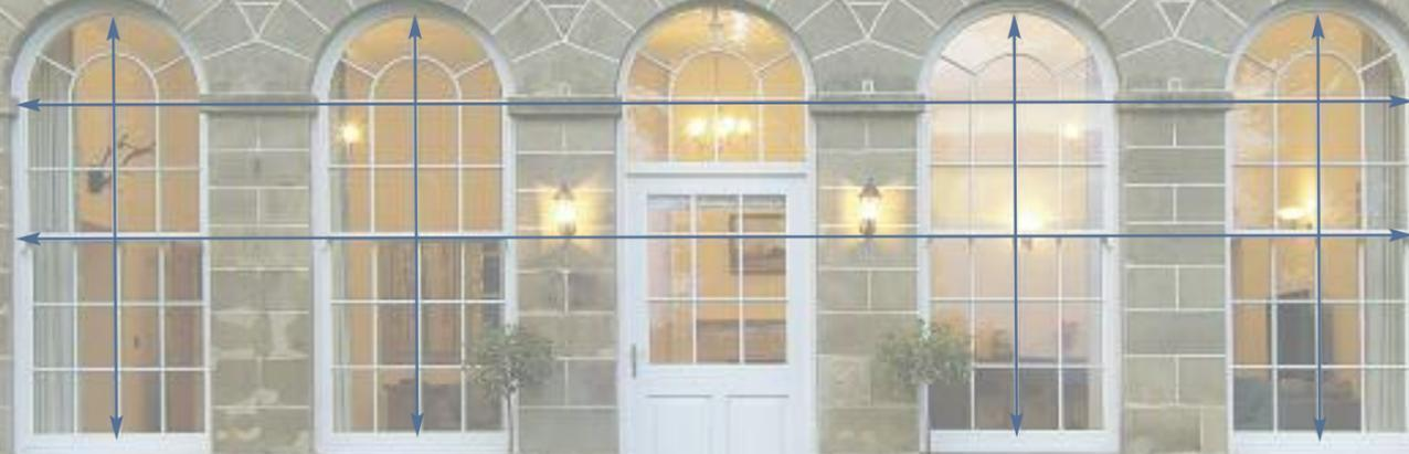
Well-thought out sightlines can make all the difference to the visual impact of your home. Wherever possible, the horizontal lines formed by window bars should match up across the windows and doors of the property. The annotated illustration above shows this design 'trick' more clearly.
