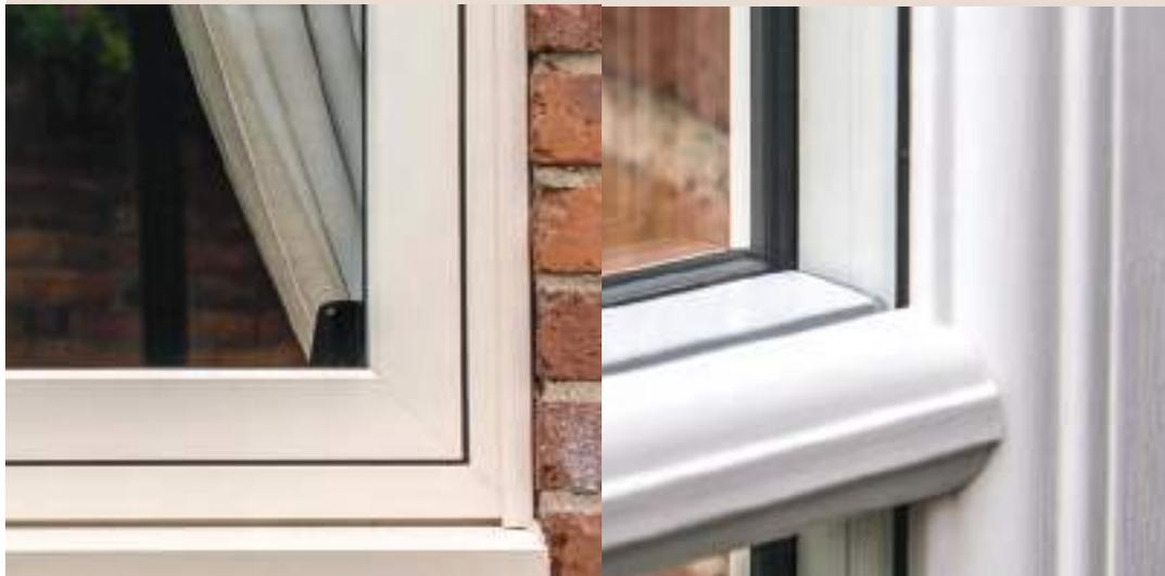
Welded joints on both outer frame and Flush Sash
