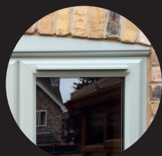
Trickle vent through a Rebated Sash
