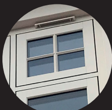
Trickle vent through the Flush Sash outer frame
