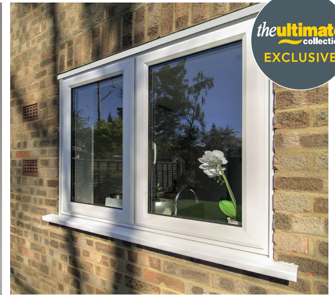
Concealed Ventilation installed through the outer frame
