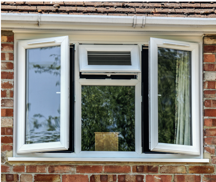
Trickle Vents installed through the window sashes
