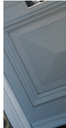
Envelope panel with Bolection Moulding
