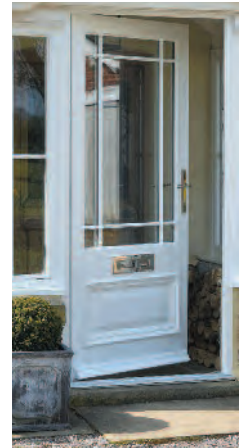
Raised and Fielded panel with Belection Moulding
