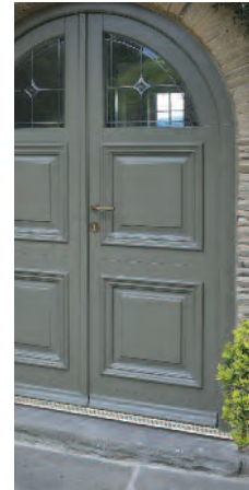
Raised and Fielded panel with Belection Moulding
