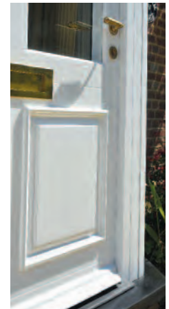
Raised and Fielded with Putty Bolection Moulding – Listed Range
