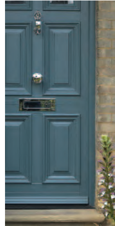
Raised and Fielded panel with Belection Moulding
